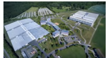
WITTENSTEIN SE headquarters in Igersheim-Harthausen
