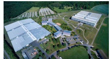
WITTENSTEIN SE headquarters in Igersheim-Harthausen
